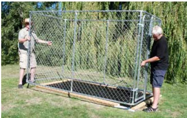
**14** Your freestanding kennel can now be placed on top of the kennel floor frame assembly and anchored in place by drilling holes in the bottom rail of the kennel and installing 3" screws through the rail and into the frame. If you are planning to install any accessories inside the kennel that won't fit through the kennel door, be sure to put them on the floor and lift the kennel over them before securing the kennel to the floor frame assembly.
