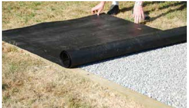
**10** Staple one corner of the kennel floor to the frame using several staples placed close together, then pull the opposite corner as tightly as possible and staple it in the same manner. Repeat this process for the remaining corners. Install staples every 4" on all sides of the floor while pulling the edges towards the outside of the frame. Trim any overhang with a razor knife or heavy duty scissors.
