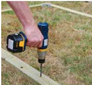
**4** In preparation for securing the frame to the ground, drill 1/2" diameter holes (8 altogether) at each corner and midway along each side of the frame.
