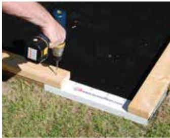
The corner joints of the top frame should criss-cross the corner joints of the bottom frame for added strength. With all the top frame pieces cut to length, determine which one will cover the scupper and cut off 12".
