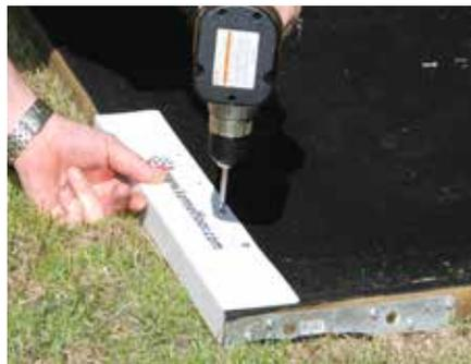
**11** Position the wash-down scupper at the lowest corner of the kennel floor platform, flush with the edge. Screw it down
