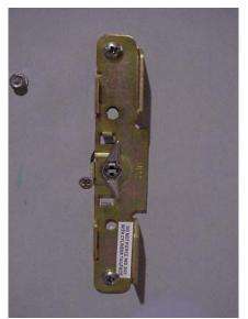
Install Detex subassembly on inside of gate using two 1/4" x 1" Install exit bar as shown in other long screws, into lever handle assembly.
