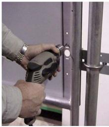
Install adjustable mounting plate onto gate. Drill hole to allow for wiring from control trim handle
