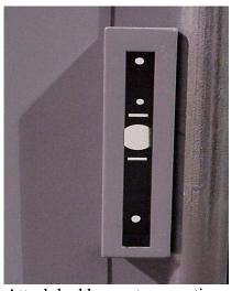
Attach lockbox onto mounting plate using two countersunk screws.
