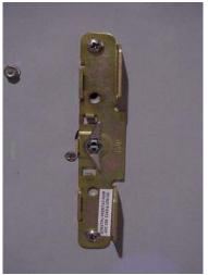
Install Detex subassembly on inside of gate using two 1/4" x 1" long machine screws into lever assembly. **NOTE**: Cylinder tail piece must *not* extend past movable cam piece on subassembly.
