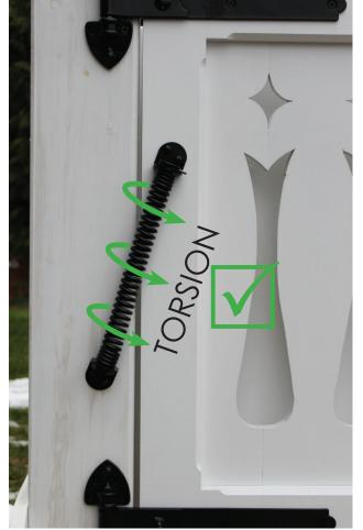
The Brutus Gate Spring is designed to apply a "torsion" force to your gate and close it. It is meant to be wound to apply force and not stretched. This means that when installed correctly, as pictured above, the act of opening the gate will further wind and/or twist the spring. When you let go of the gate the spring will want to return to its resting position.
