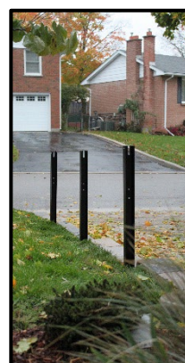
Posts installed Top Notches aligned
