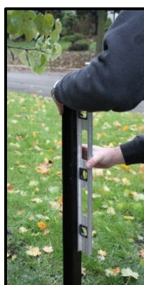
Height & Alignment Check
