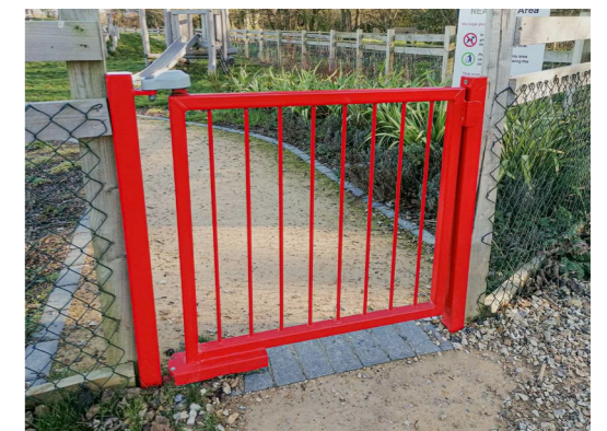
APSSTOP shown in gate
