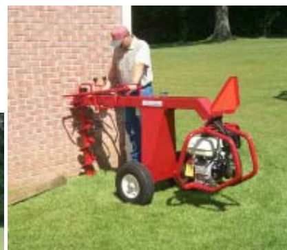
Figure 11B Up-close Drilling
