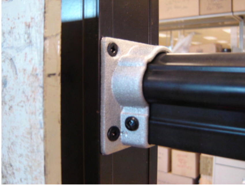
Photo No. 7 Cast Aluminum Bracket for Top Rail
