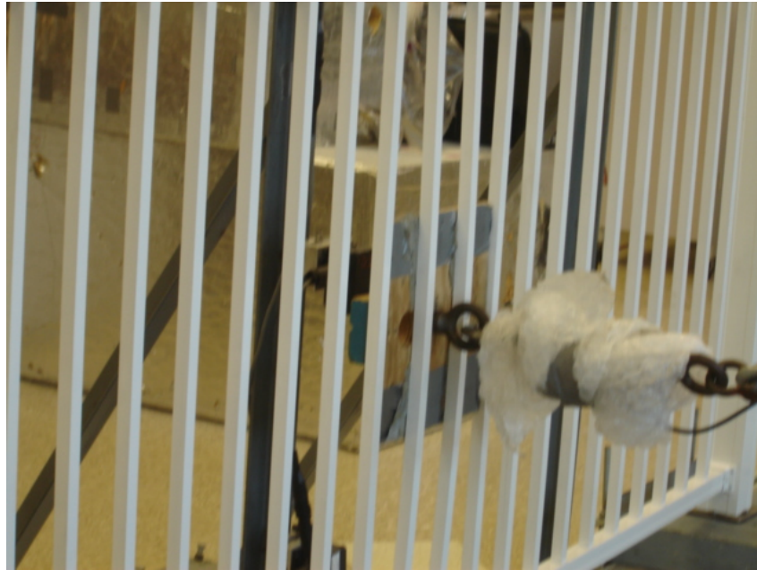
Photo No. 1 In-Fill Load Test -Middle of Baluster
