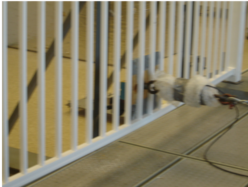
Photo No. 2 In-Fill Load Test- Bottom of Baluster
