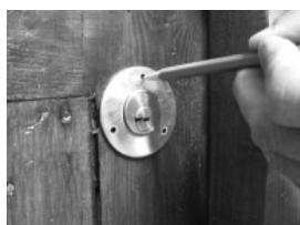
7. Fit the escutcheon plate on the other side of the gate. First hold it in place, and mark out the pilot holes.
