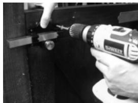
6. Put the lock back into position, and fix to the gate using the square head Philips screws, and the Philips driver bit. Once all screws are tight test the lock and ensure it turns ok- if the face of the gate is not exactly flat the lock may bind and stop it from working. If this happens you need to loosen off the appropriate screws, or insert packers until the barrel turns freely.
