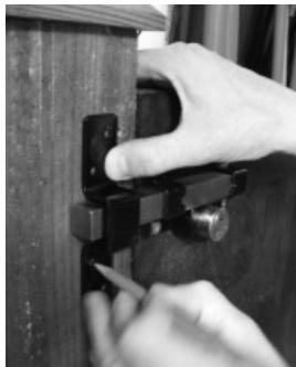
9. Fitting the keep. In this situation it is going on the gate post. Turn the lock to the locked position, and place the keep over the top of the bolt, allowing sufficient room for gate sag over time. Line it up straight with the edge of the gate post, and mark through the holes for drilling the pilot holes in the timber.
