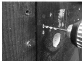
5. Drill your pilot holes in the gate with the 3mm drill bit.
