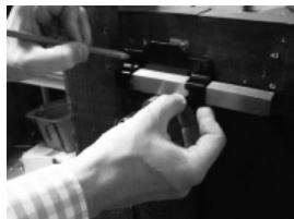
4. Now insert the lock into the hole, and test to ensure the lock will work in the situation. If it is OK level it up in line with the edge of the gate, and make marks through the fixing holes for the pilot holes.
