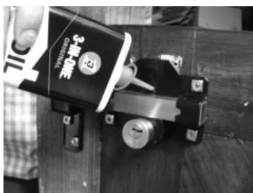
11. To ensure a long life from the lock you must put oil down between the bolt and the back plate at least once every 3 months - if it is situated in a coastal area, or in a high use situation, then this must be done at least every month.
