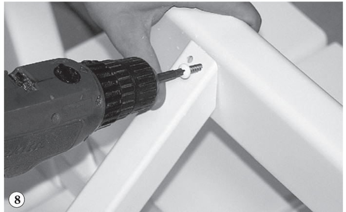
8 Secure the brace to the beam with screws.
