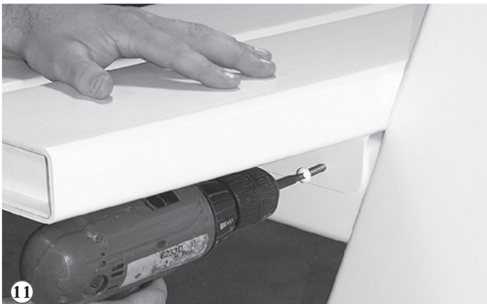
11 Place the benches on the beams and fasten in place with screws, as shown. Your table is now complete. Enjoy!
