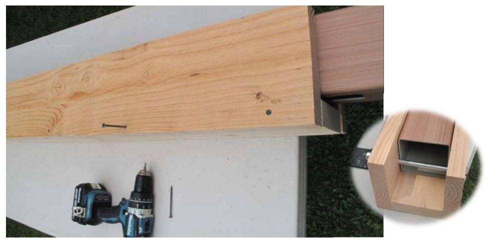
For best results, pre-drill and countersink screws through the side pieces into the base.
