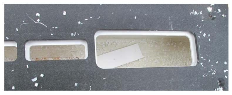
Loosen template and slide up post until last 7/8" x 3" hole cut-out is centered on post
