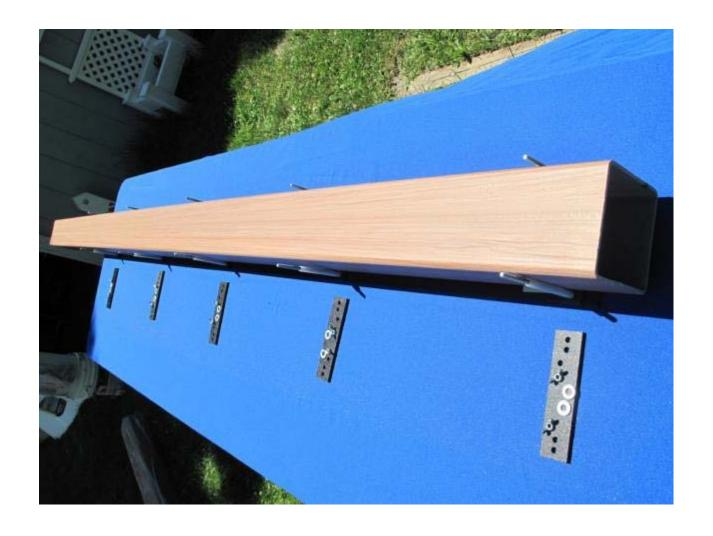
Lay post face down on template with measured hole facing down. Finish assembling the clamping plates and hardware. Install but do not tighten bolts.
