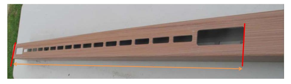
Measure from top of post to bottom of 2 x 6 cut out.
