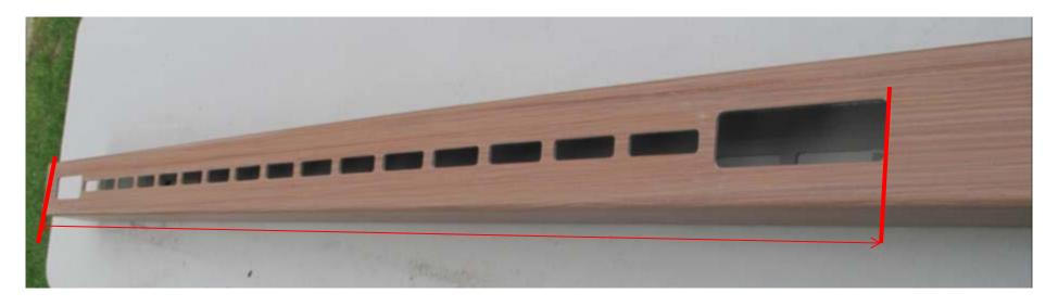
Measure down from top of routed post to bottom of 2 x 6 hole Example 75"
