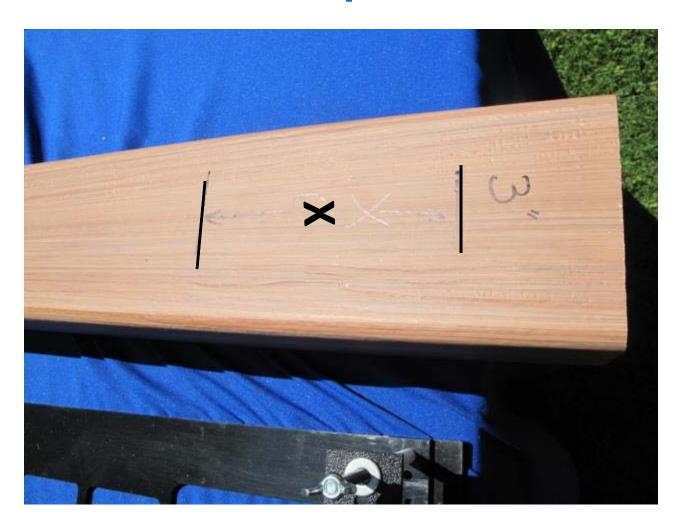
Mark post - measure down 3" from top of post Mark post with 6" long hole- indicate with X in center
