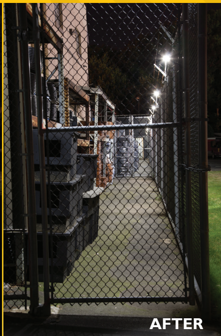
For Fence Perimeters: CAST LED Perimeter Fence Light (CPL1)
