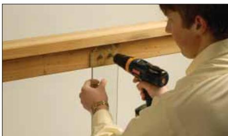
**Step 2:** Attach the first baluster on-center of the center line using four of the screws provided. Drive each screw until the rubber grommet begins to mushroom. Do not over-tighten.
