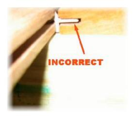
The lower portion of the groove must be pushed slightly down to the joist by the short point of the fastener. The pressure downward on the groove should be light to moderate. The decking should not be loose or floating under the short point of the fastener, readjust until the back edge of decking is snug.
