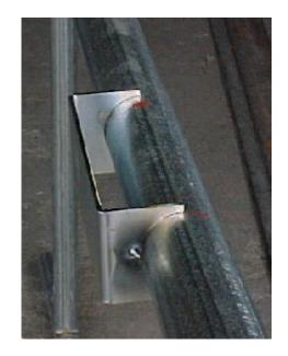
Step 1: Align and tack weld our SHUT IT HardCORE Carriage Cap (CI2340 or CI2360) on top of your bottom rail.
