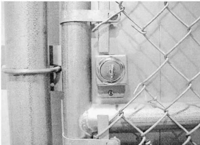
13. After latch bracket is adjusted properly, attach to post with tek-screws.
