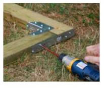
In preparation for securing the frame to the ground, drill 1/2" diameter holes (8 altogether) at each corner and midway along each side of the frame.
