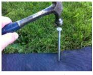
the Perfect Kennel Floor tight enough so it lays flat and smoothes out any creases and drive in another spike. Repeat for the two remaining corners and then install the rest of the spikes evenly around the perimeter of the floor, remembering to stay back approximately 2" from the edge of the material.
