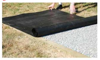
Staple one corner of the kennel floor to the frame using several staples placed close together, then pull the opposite corner as tightly as possible and staple it in the same
