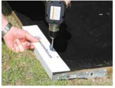
Position the wash-down scupper at the lowest corner of the kennel floor platform, flush with the edge. Screw it down
