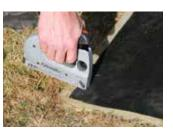
manner. Repeat this process for the remaining corners. Install staples every 4" on all sides of the floor while pulling the edges towards the outside of the frame. Trim any overhang with a razor knife or heavy duty scissors.
