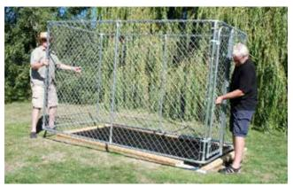
Your freestanding kennel can now be placed on top of the kennel floor frame assembly and anchored in place by drilling holes in the bottom rail of the kennel and installing 3" screws through
