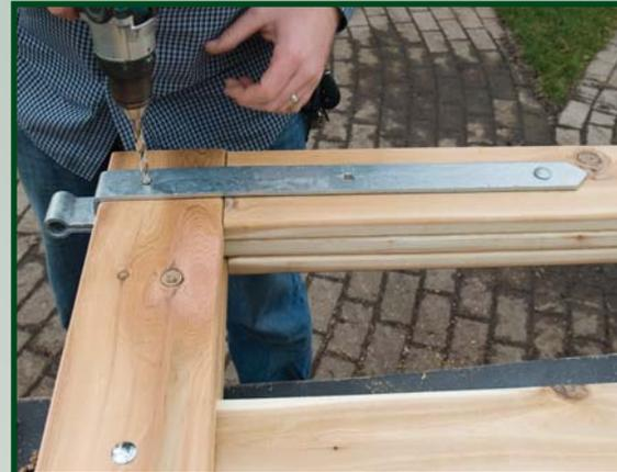
**10** When installing bolts do not install bolts at top corner where hardware will attach. Center hardware on rails, drill holes and attach with fasteners provided.
