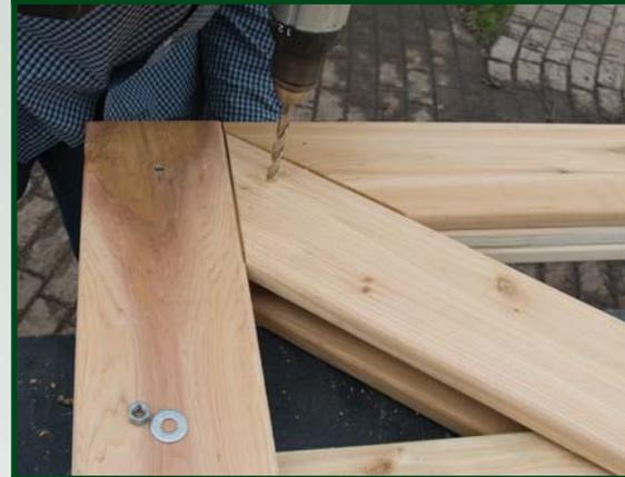
**9** Turn the gate over and repeat steps 5 thru 8 on the other side. Drill a hole at each intersection point and install 3.5" x 3/8" galvanized carriage bolt at each location.
