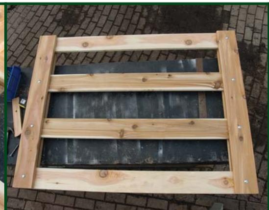
**5** Measure distance between stiles and cut upper rail to fit. Place in position but do not fasten at this stage.
