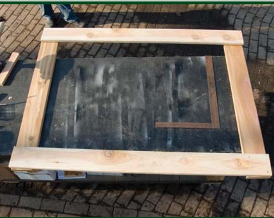
**1** Lay out two vertical risers (stiles), to rail and bottom rail in rectangular shape. Fasten each of the outside corners with a single 1.5" wood screw.
