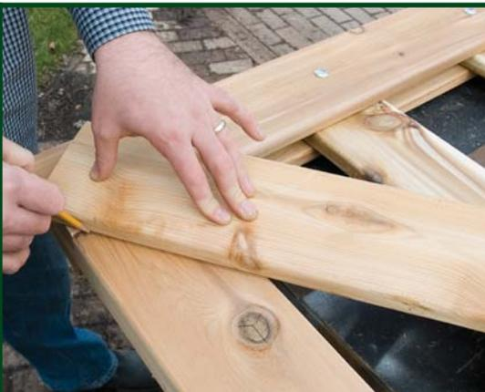
**6** Lay diagonal braces on surface (allow 1/2" from top of top rail) Mark top rail with pencil line.
