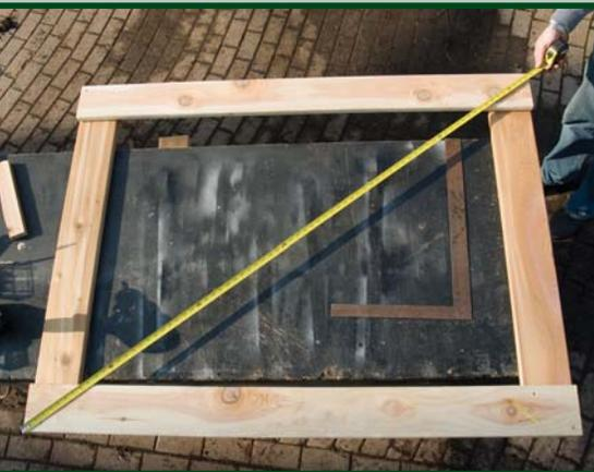
**2** Measure the two diagonals and adjust gate so that they are equal (this will ensure the gate is square). Install another 1.5" fastener at each inside corner.
