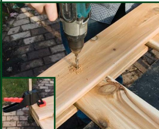
**4** Turn the gate over. Attach second stile at each end. Use 3.5" x 3/8" galvanized carriage bolts. Tip: use quick clamps to hold stiles in place while drilling.
