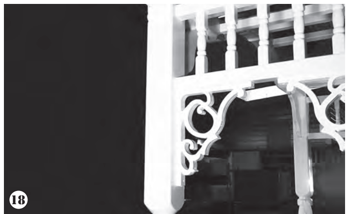
18 The scroll is fitted over the starter strip and secured in place with screws.
