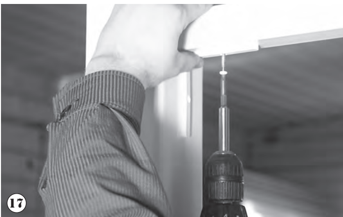
17 Gingerbread scroll starter strips are screwed into place centered on the bottom of the upper railing assembly and the post.
