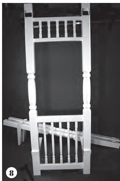
8 Finished, a side wall is ready to be put into the arbor. Notice how the post is routed to accommodate the railing and roof sub assemblies, especially the corner braces. See Figs #12 & #13 for more information in determining post orientation. Having the posts orientated correctly when beginning the assembly is required.
