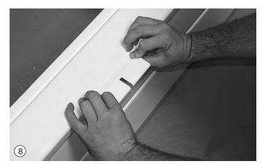
Position the lid latch at the center of the front of the lid, predrill and screw in place.
